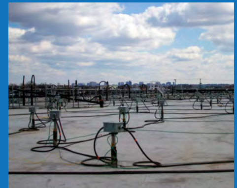
Well field during thermal conduction heating operations
