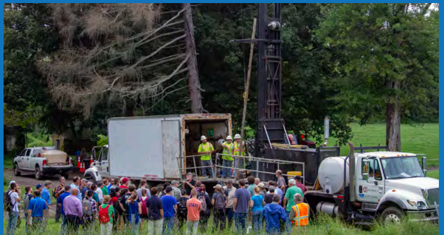
Cascade Drilling, with the Midwest Geosciences Group, collecting samples and demonstrating sonic coring techniques as part of a workshop entitled, "Managing the Complexities and Uncertainties of Soil Sequences" in West Chester University, PA.
