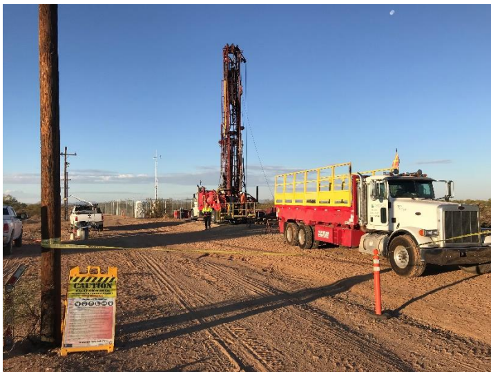
Drill site setup with 50K drill and support truck
