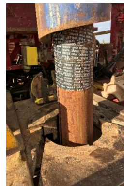
Drop pipe & column pipe retrieved from the existing wells
