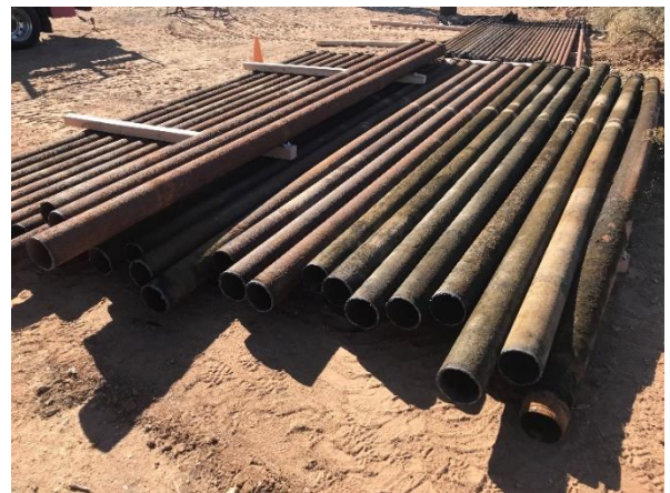
Drop pipe & column pipe retrieved from the existing wells
