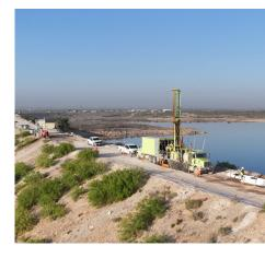
However, the sensitivity of the embankment meant traditional drilling methods could entail unacceptable risks, including damage to the structure or uncontrolled material loss. The client needed a precision drilling solution that would protect the dam while supporting the installation of a subsurface seepage barrier.
