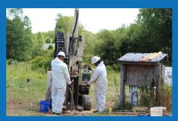
Cascade Technical Services crews provide calculated injections to remediate soil and groundwater contamination
