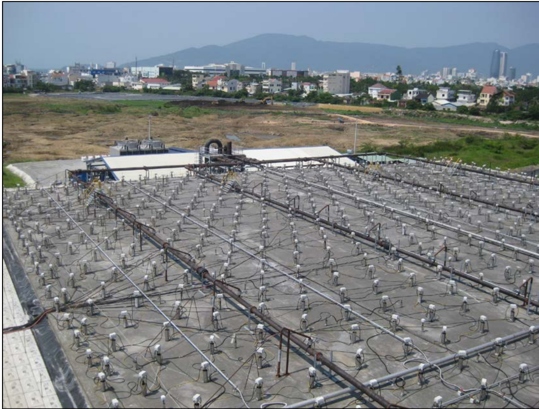
In-Pile Thermal Desorption (USAID- Danang Vietnam)
